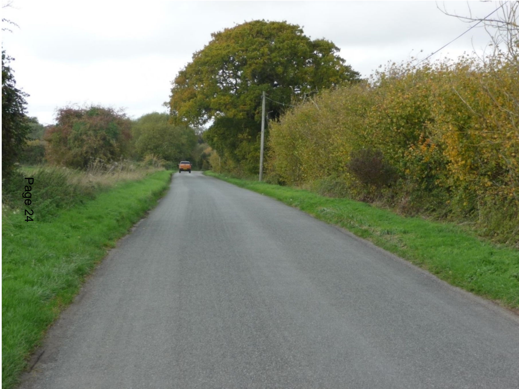
COATE ROAD (SITE ON RIGHT HAND SIDE)
